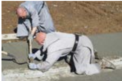
As more trucks arrive, monks and volunteers work together to finish pouring the concrete foundations for several new buildings.
